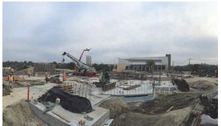
Walls are going up! A view on March 19.
