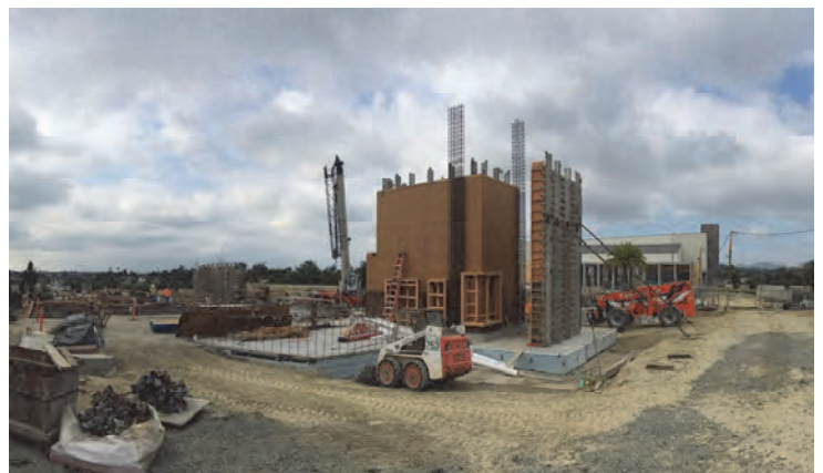
The base of the tower A view on March 25
