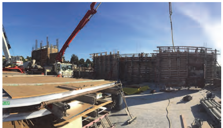
Pouring concrete walls A view on April 3
