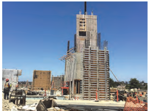
Forms for the next level of the tower!
