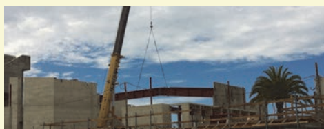
Setting one of the roof beams in place.
